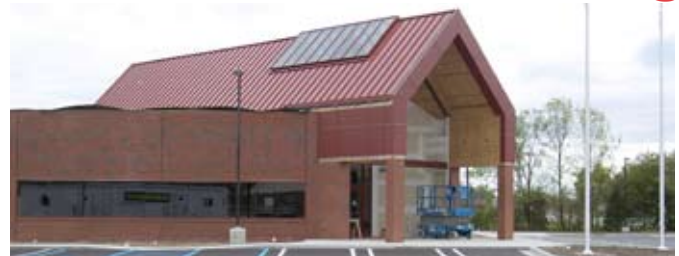
Communications Family Credit Union Branch Office - Midland RC Hendrick & Son Construction built this beautiful new office for CFCU located at 100 Joseph Dr. in Midland. A!BM was contracted to clean all the glass including skylights, strip, seal and refinish all the vinyl composition floors, clean the ceramic grout in the lobby, wipe all surfaces and clean & sanitize the restrooms.
